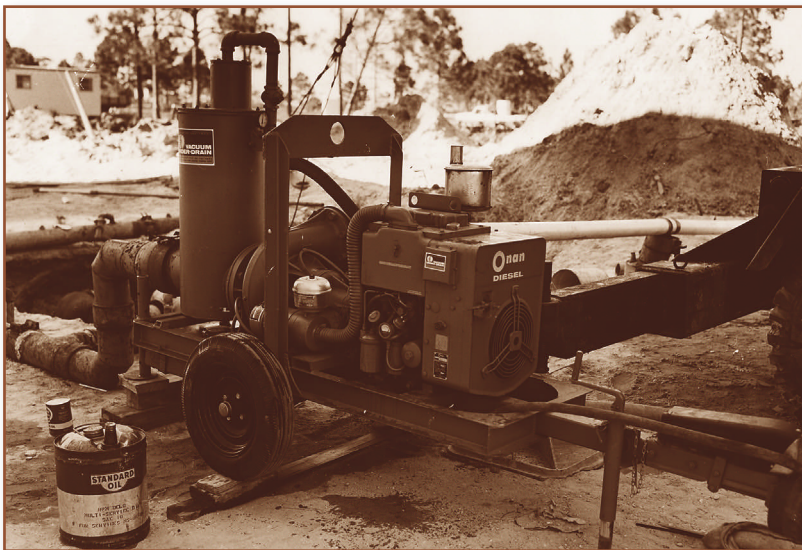
In 1973, Thompson adapted the rotary pump for wellpoint dewatering — the first time a rotary pump had been used for that application.
